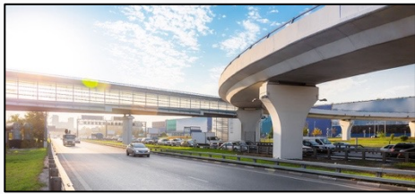
Efficient operation and management of critical social infrastructure
