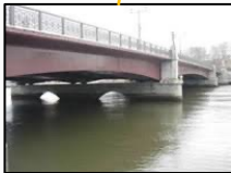
Bridge strain monitoring.
